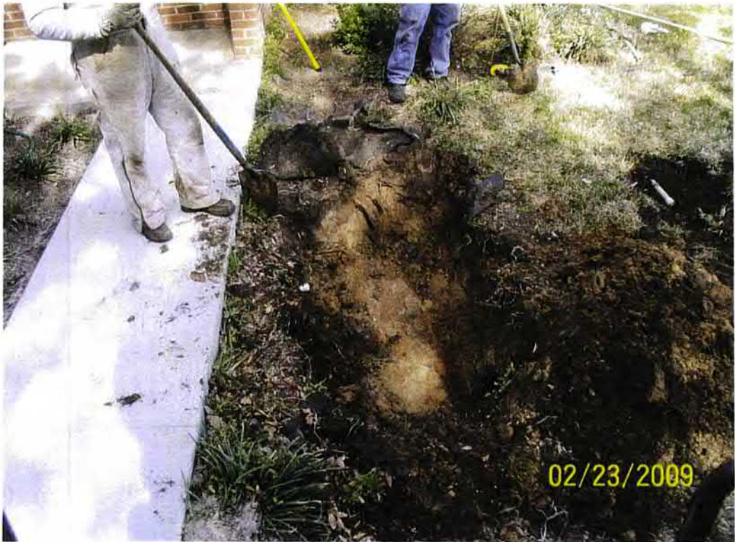
Picture 2: UST 129 Banyan-2 during removal.
