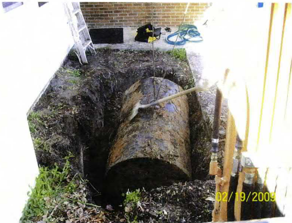
Picture 2: UST 129 Banyan-1 during removal.
